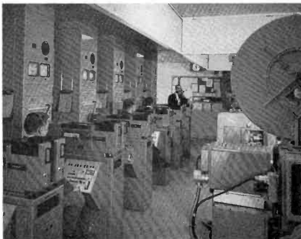
Film programs originate in the 'telecine area,' which also handles film inserts in live programs for the CBS-TV network and WCBS-TV New York. A bank of slide projectors is at the left and a film projector is at the right.
